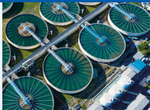
Decentralised data acquisition
